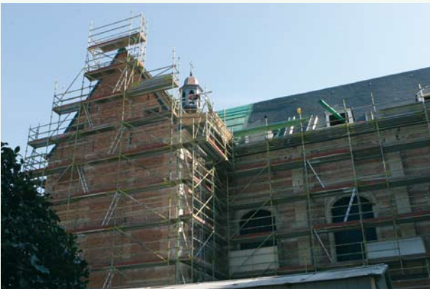
Renovation of the convent
